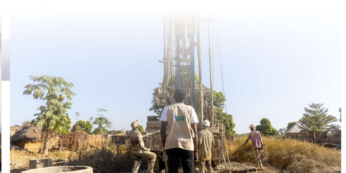
Zion during an on-site monitoring of borehole drilling/construction.
